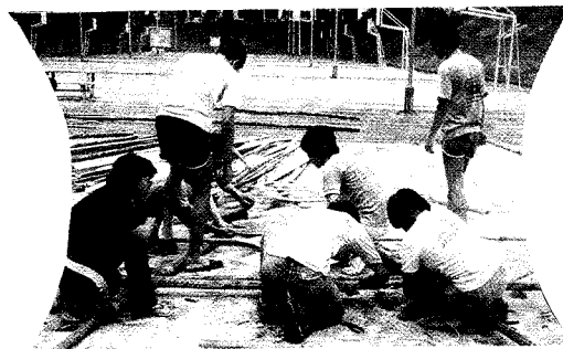
Building the gate
